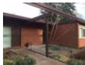
Finished beam and support column
